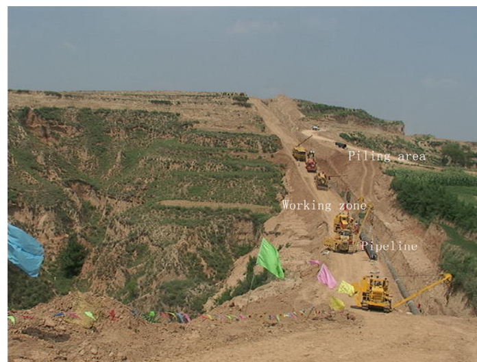
Figure 2. Pipeline right-of-way including trench, piling area and working zone.
